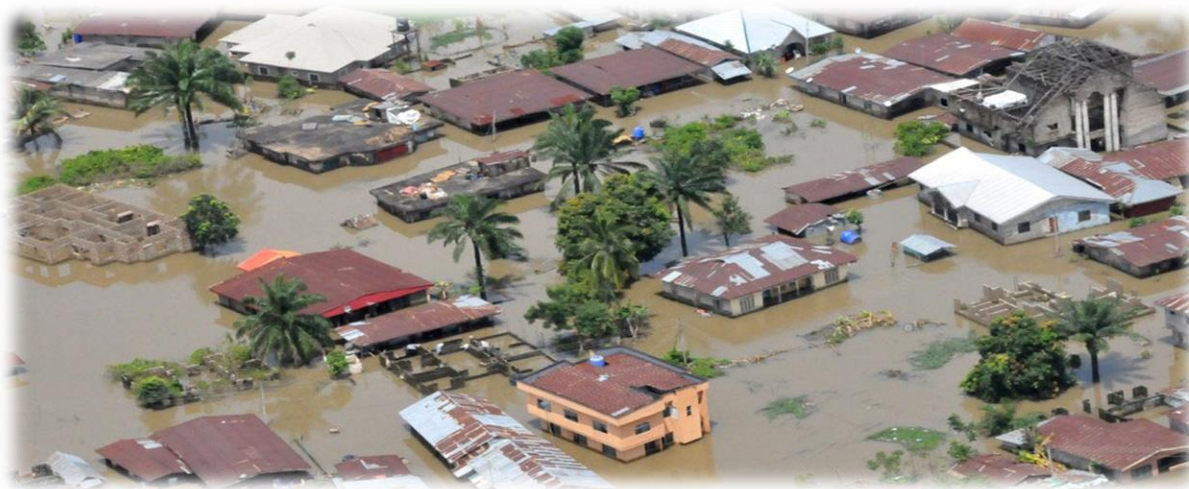
Figure 4: Houses destroyed by flood
