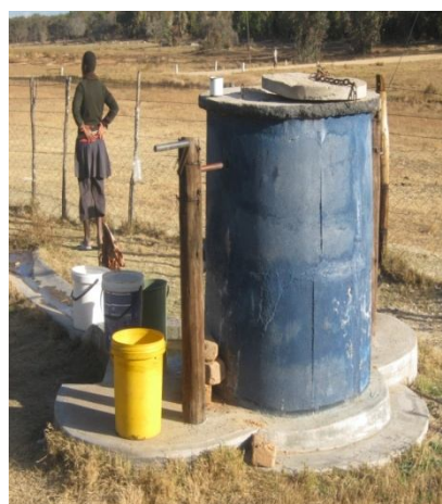
Plate 4 The borehole in Tapfuma garden constructed with Caritas assistance
