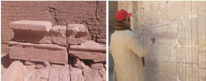
(Figure.3) Obliteration of engravings and climate impact on constructional sandstone of Dush temple
