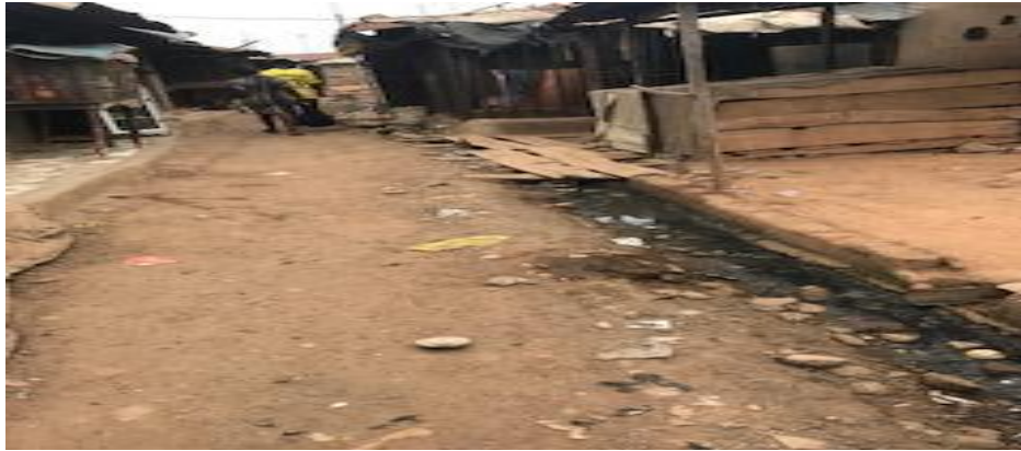
Plate 2: Gutter and Drainage Littered with Waste in Jabi Main Source: Fieldwork (2018)
