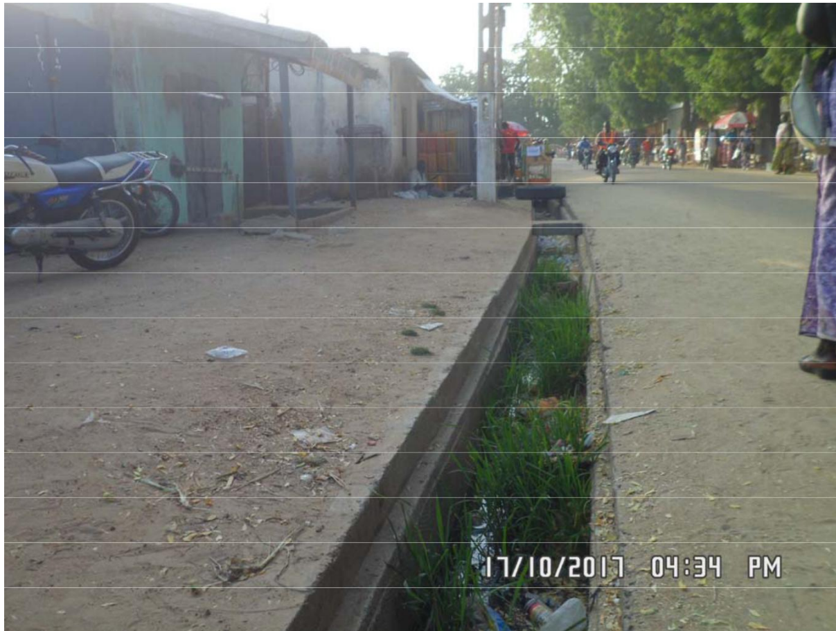
Photo 2: Non-cleaning of rainwater drainage pathways
